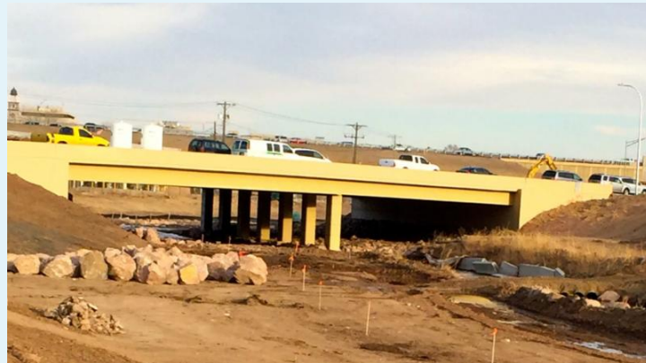
US 24 Bridge Over Upper Fountain Creek
